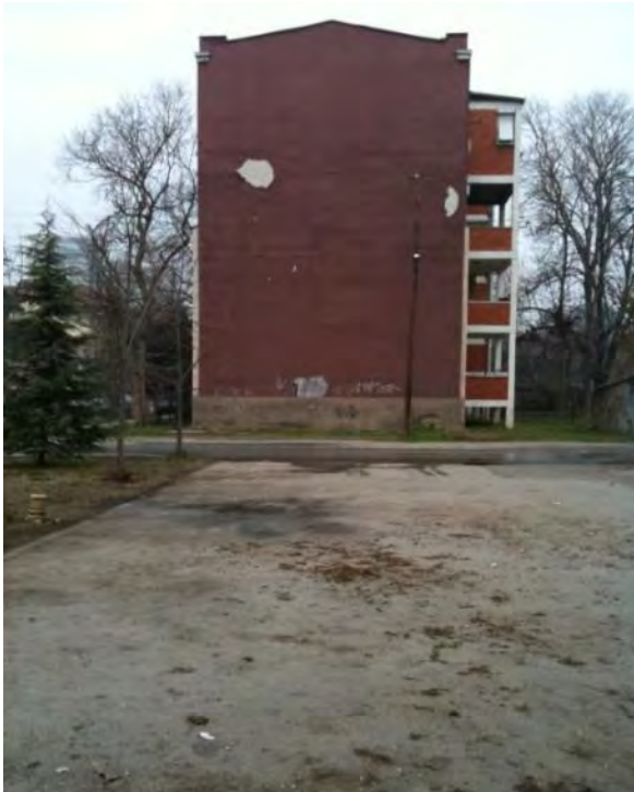
Fig. 5. Building + enlargement, "Prolet" settlement, 2013.
